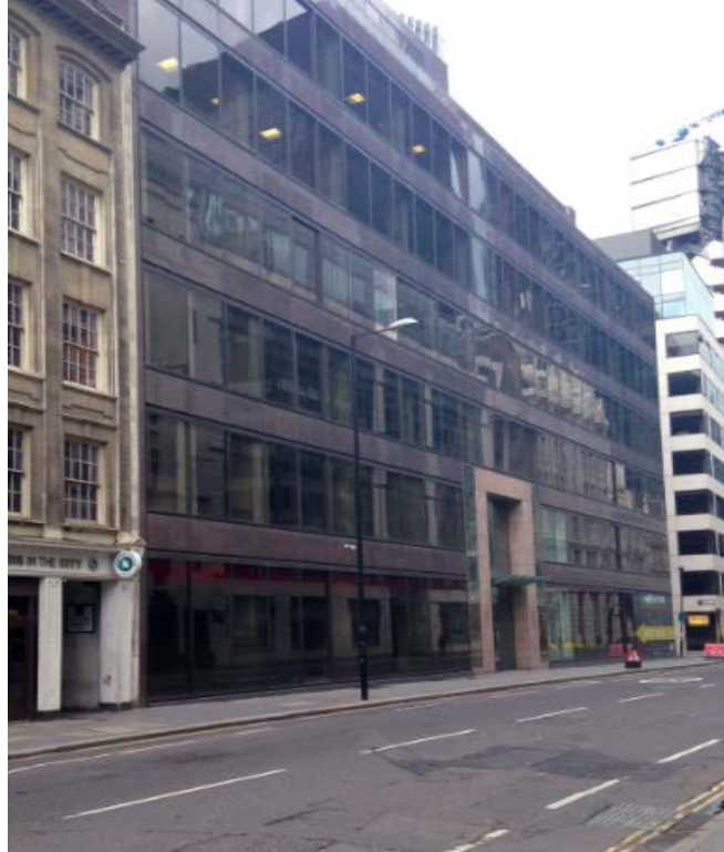
Figure 3.1. 44-46 Leadenhall Street London former site of the African House, headquarters of the Royal African Company. Sometime between 1752 and 1766 when company officials met at Cooper's Court in Cornhill, the original building was pulled down. A 1745 account stated that the "Royal African-house is situated on the south side of Leadenhall Street, near the east end of it. Here the affairs of the company are transacted but the house has nothing in it that merits a particular description." Thomas Osborne, A Collection of Voyages and Travels (London: T. Osborne, 1745), 116. Photograph by Neal Polhemus, 2015.
